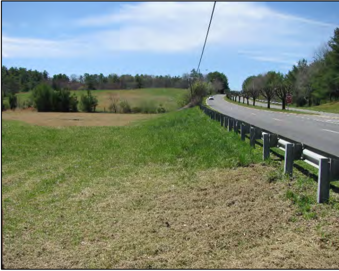
Existing Route 58 Entrance – Looking West
