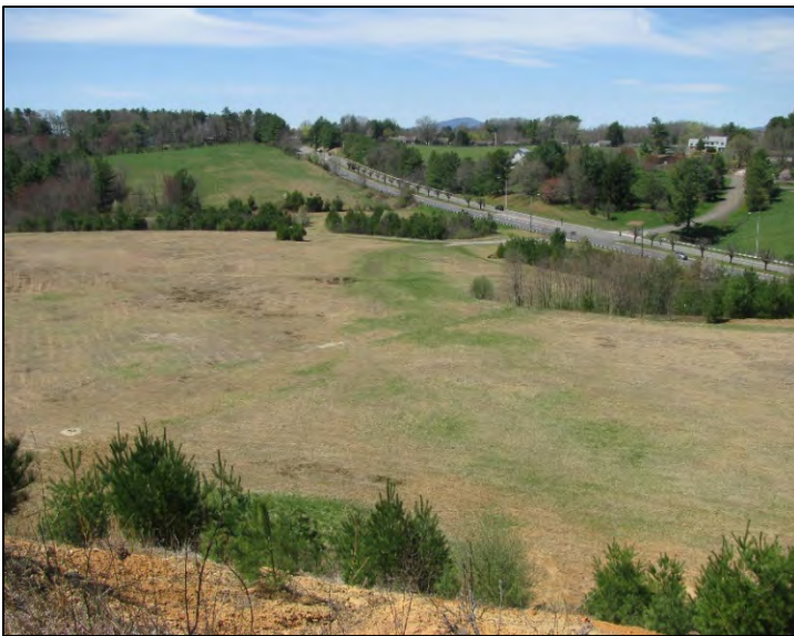
Graded Route 58 Frontage
